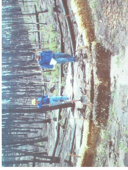
**Contour felling of small diameter trees on slopes, and tree trunks and straw bales in swales are inexpensive and effective erosion controls.**
